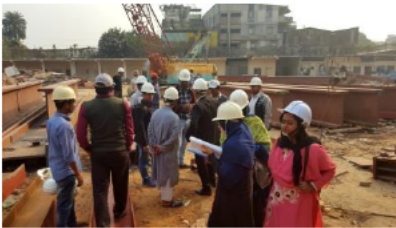
The group went to the field to inspect the lifting equipment in the real world
